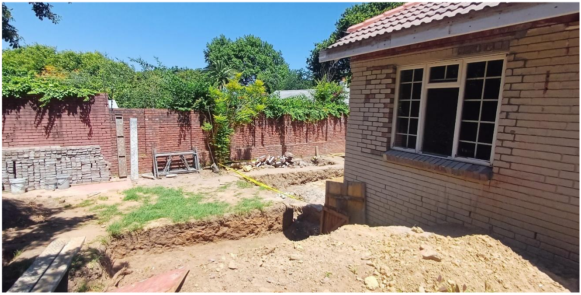
Figure 32: The back garden of the study property showing initial excavations.
