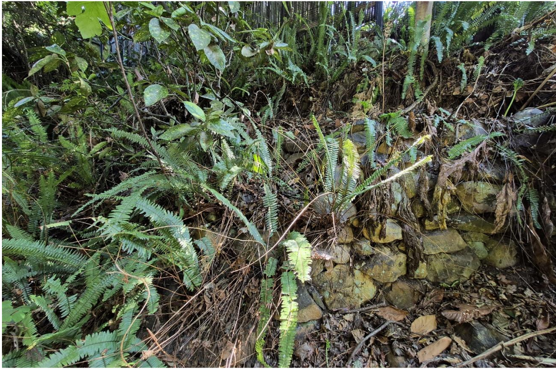
Figure 43: Retaining wall made of river boulders, on the north bank of the stream.
