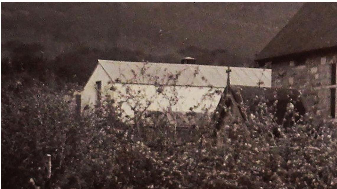
Figure 10b: Detail of the same image showing the long building. Here a loft door and corrugated iron roof can be seen, along with what seems to be a roof vent. These features could be consistent with a stable, although what appears to be a low veranda is partially visible, indicating a possible conversion into a dwelling (the 1927 street directory lists unnamed Coloured people living there).
