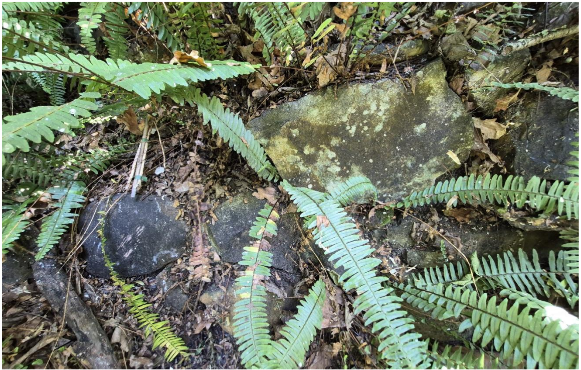
Figure 42: Retaining wall made of river boulders on the north (graveyard side) bank of the stream.
