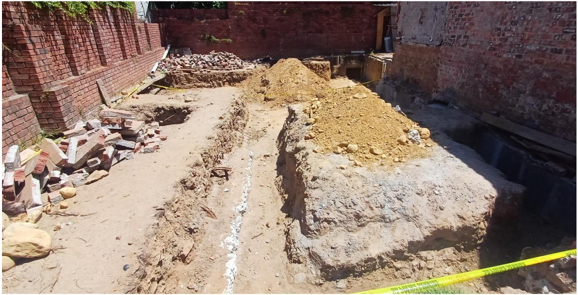
Figure 36: Looking approximately south down one of the trenches.
