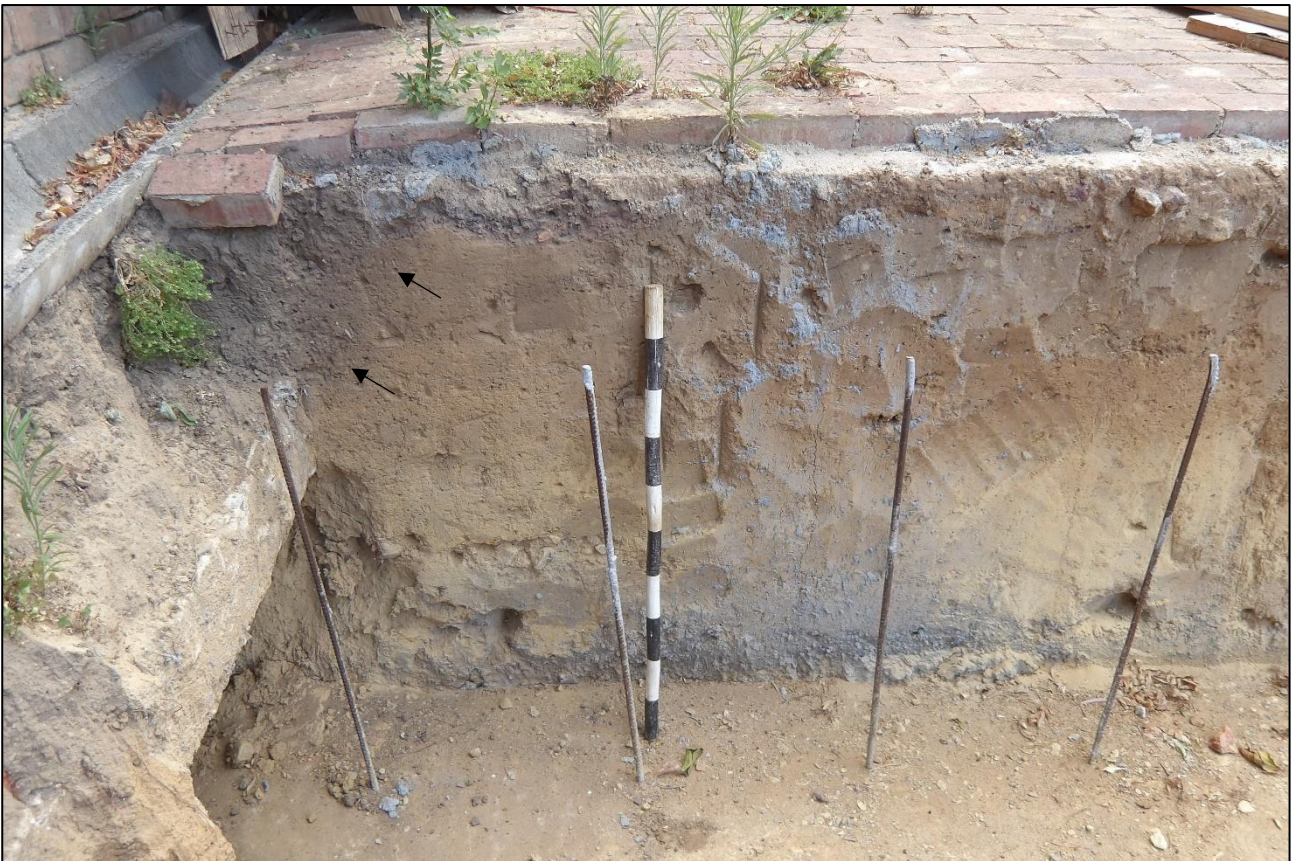
Figure 8: Looking towards the northwest at the section at “A”. The ranging rod rests on the newly cast foundation. The foundation of the boundary wall to the southwest of the site is visible to the left and its trench cut (now bioturbated) is arrowed. Scale in 10 cm intervals.
