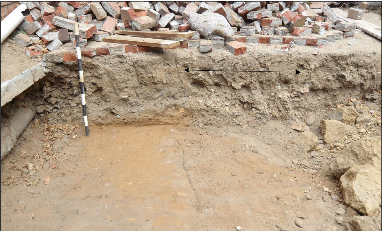
Figure 10: Looking towards the south west at the section at “C”. The arrow indicates the width of a trench that has been backfilled, while the line in the sand at the base indicates the edge of this trench extending towards the camera. Scale in 10 cm intervals.
