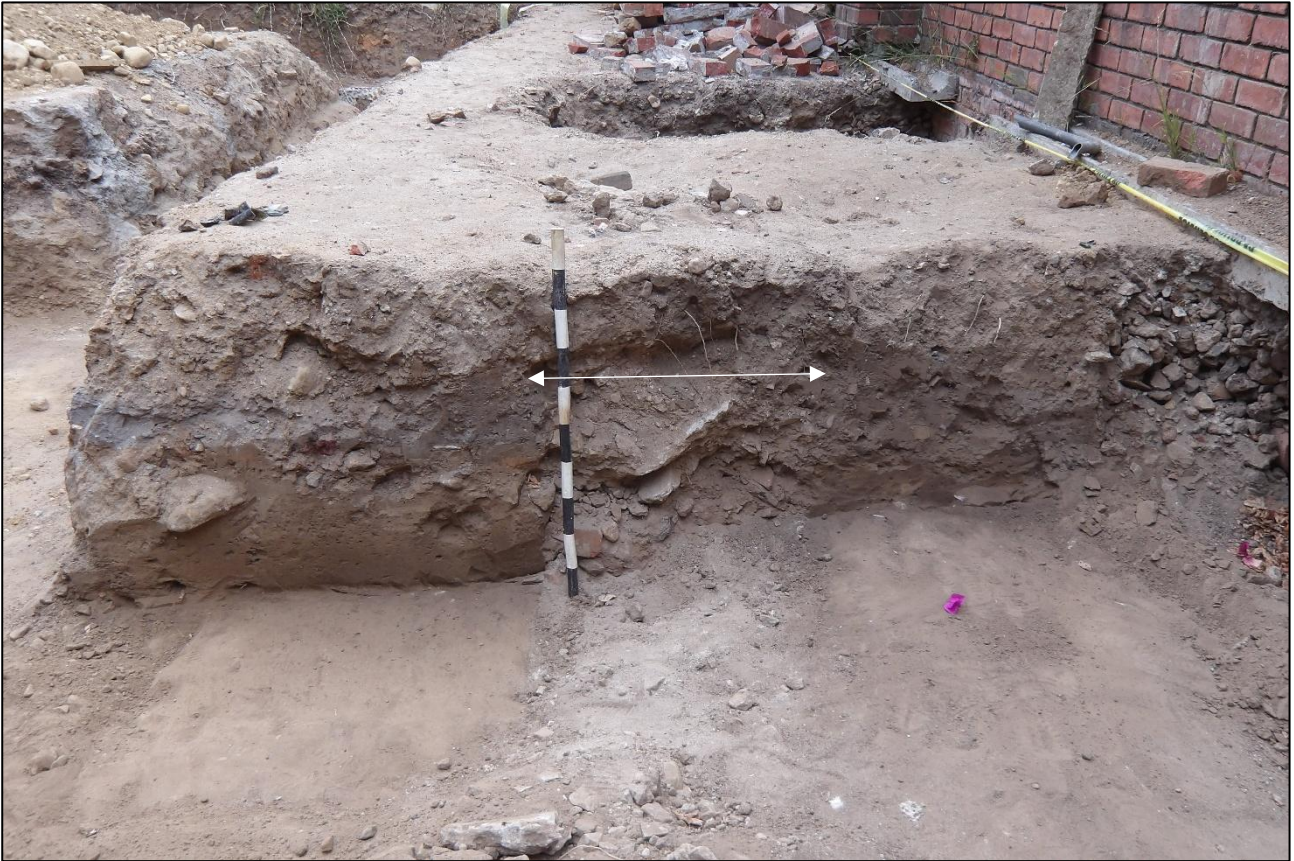
Figure 12: Looking towards the northeast at the section at “D”. A trench through this area is marked by the arrow and it is easily evident on the floor of the excavation as well. Scale in 10 cm intervals.
