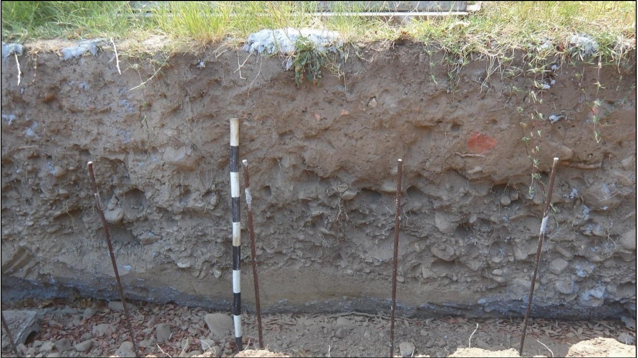
Figure 21: View towards the northwest of the section at “H” with the base (covered in gravel and fallen leaves) being a newly cast wall foundation. Scale = 1 m.
