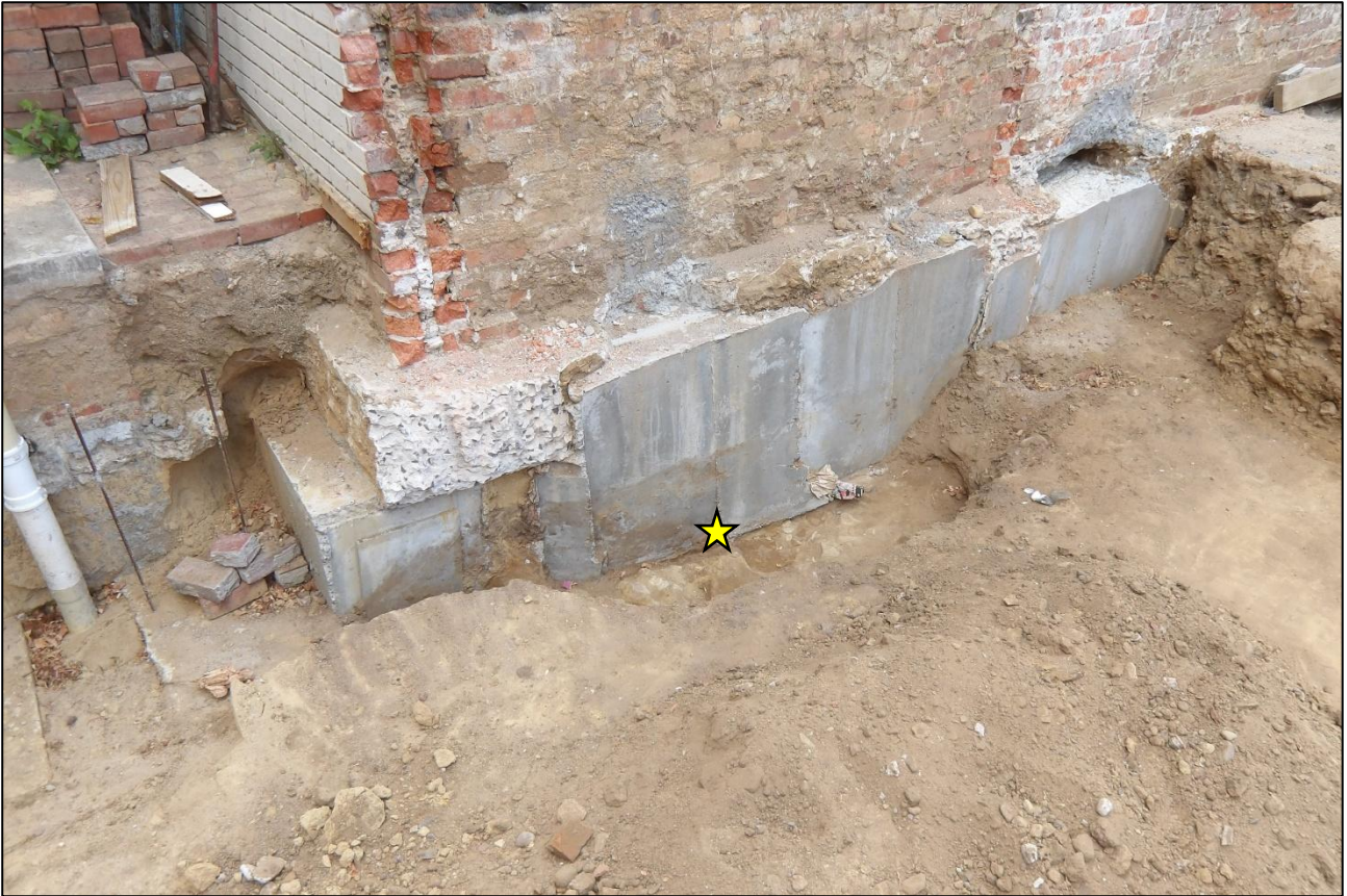
Figure 6: View of the section of the property where the human remains were found. The yellow star marks the approximate location from where the bones were recovered.
