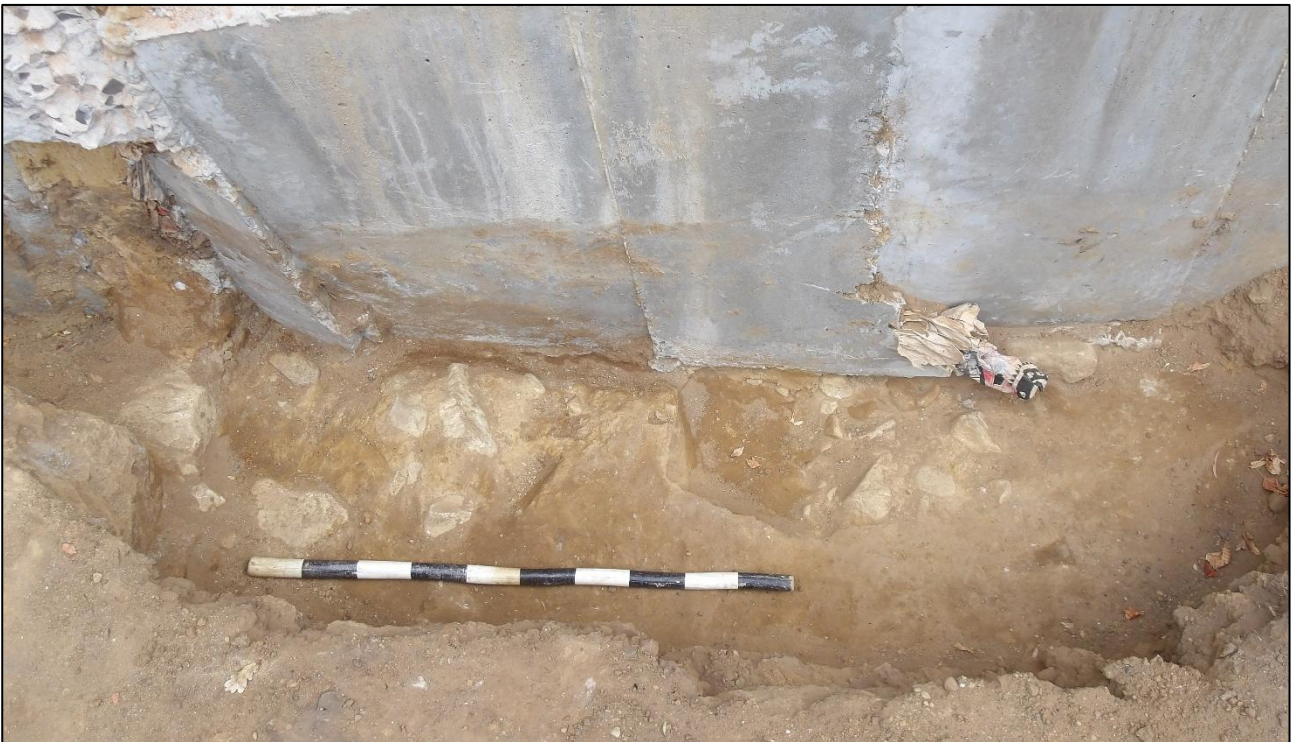
Figure 7: View into the excavated trench where the remains were found. According to the builders, they were centred on the area at the foot of the cast concrete above the 1 m scale bar.
