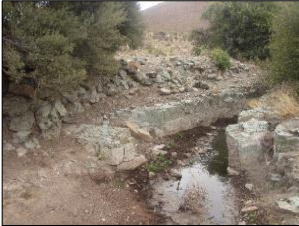
Figure 5-17: Water reservoir at waypoint HL1810.
