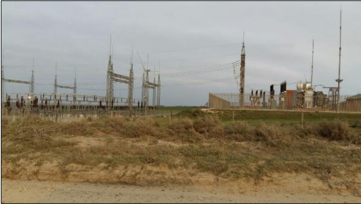
Figure 1-4: Example of an Eskom switching station (left) and adjoining Wind Farm substation (right) on the Kouga Wind Farm.
