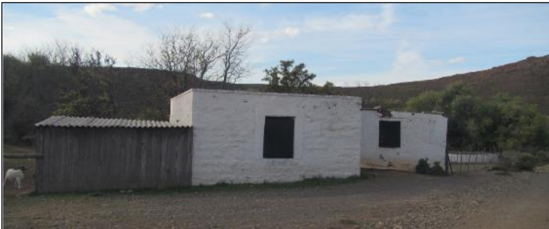
Figure 5-45: A stone-walled outbuilding within the Leeuwkloof farm complex (waypoint NV1850).
