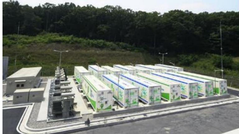
Figure 4: Example of a 15-container Lithium-Ion BESS installation
