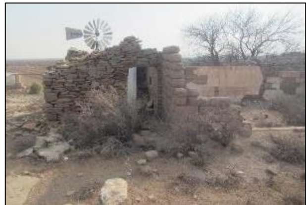
Figure 5-21: Part of a house at waypoint 112 in HL02.
